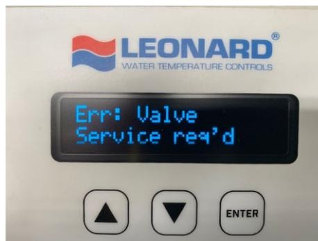
This Error indicates that the Proton Valve has reached less than 90% of initial Sweep Value recorded in Step #10. This translates into lost motion on the shuttle and ultimately loss of ideal temperature control. The Mechanical Valve Components should be taken apart, cleaned of any and all debris or scale inside the valve body, inspected and serviced. Worn components must be replaced if necessary.
