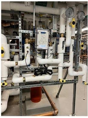
Leonard's Nucleus models give plumbing engineers complete system monitoring with outlet temperature control within +/- 2F from set point, regardless of demand. Features include user programmable set point, integral daily sweep and sanitization.
