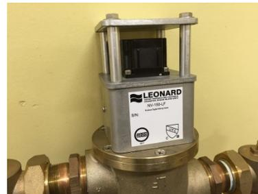
9A. **Models NV-150-LF and NV-200-LF:** First loosen the locking nut and then remove the sleeve assembly by unthreading it from the base (special tool required).
